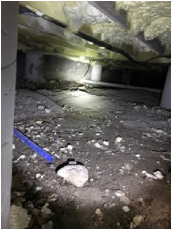
RIGHT SIDE CRAWL SPACE
