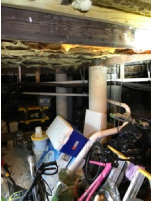
LEFT CRAWL SPACE
